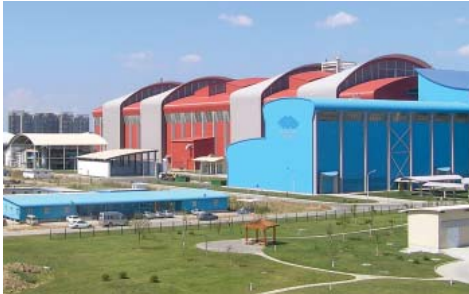
Metal coating and paintline facility BlueScope Steel, Suzhou, P.R. China
