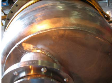
Inspection of large pressure vessel component
